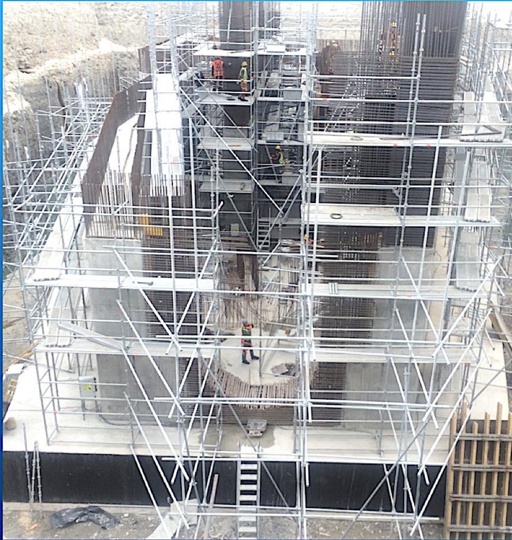
WATER INTAKE BUILDING AND DIFFUSER PORT MANUFACTURING
